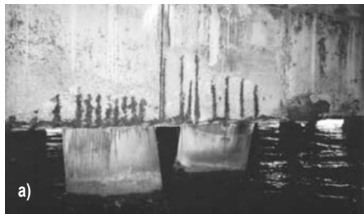
Figure 1. Examples of the effects of corrosion of steel in concrete: (a) spalling of the concrete cover due to carbonation induced corrosion, (b) localised attack on a bar due to pitting corrosion in chloride contaminated concrete.
