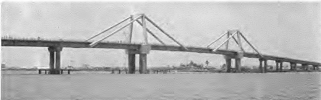
21-22-23 - The bridge over the Rio Magdalena at Barranquilla in Colombia with a total length of 1300 m and a major span of 140 m. The bridge was built in a strongly seismic area.
