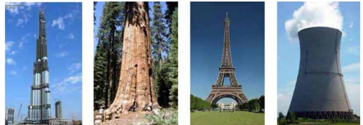
**Figure 1.** Man-made and natural uniform resistance structures
