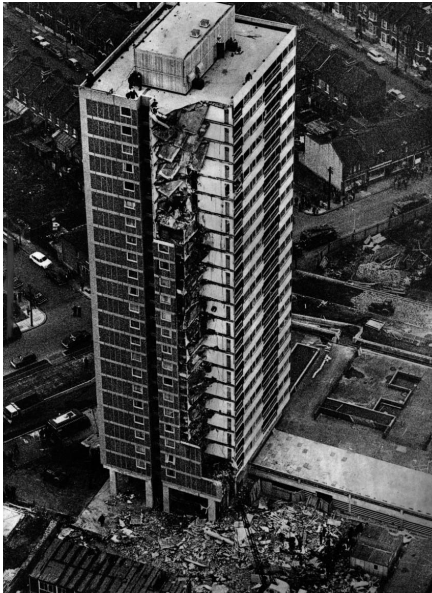
Figura 1 – Collasso Roman Point ( http://www.failedarchitecture.com/the-downfall-of-british-modernist-architecture/ )
