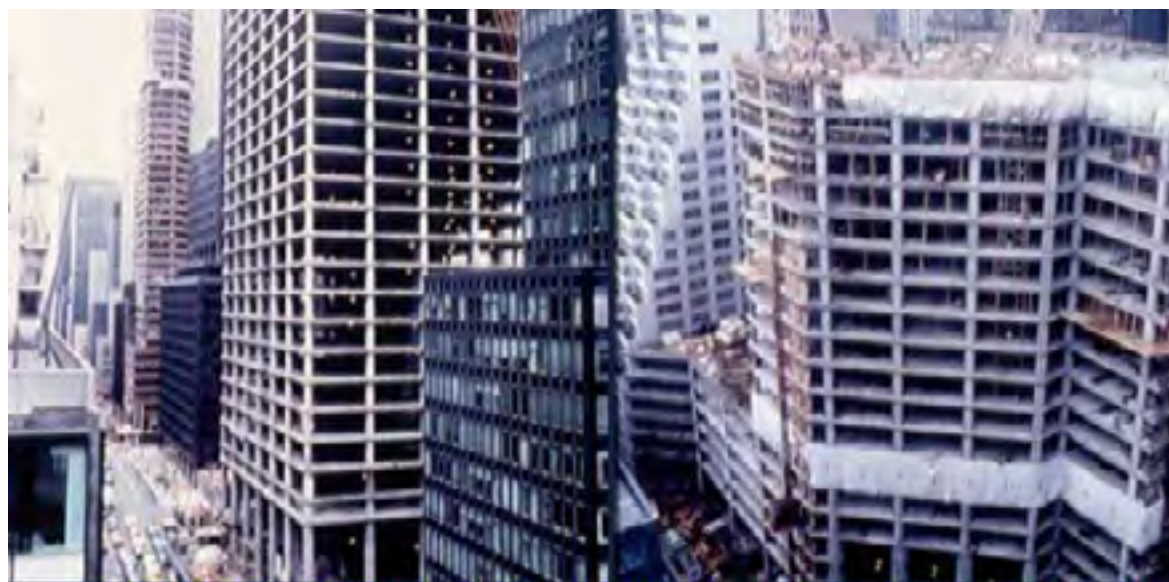
TRUMP TOWER: 1° GRATTACIELO IN CLS NEW YORK 1981 - MIX DESIGN: M.COLLEPARDI
