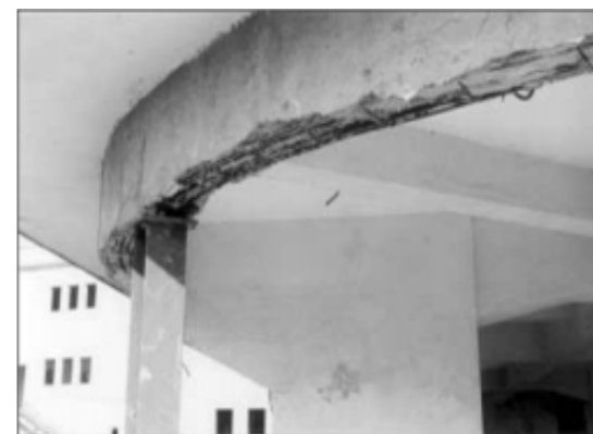
Figura 2. Trave emergente in c.a.
