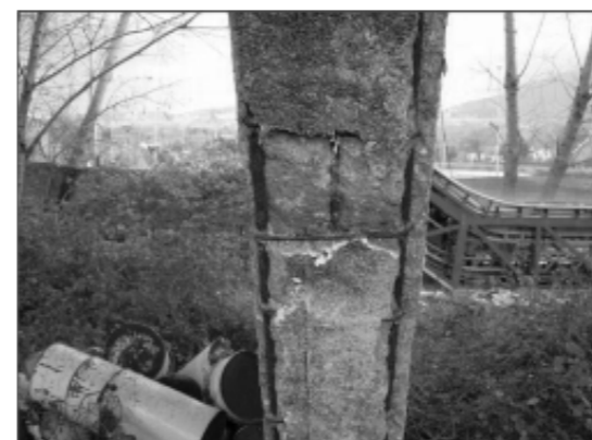
Figura 3. Pilastro in c.a.
