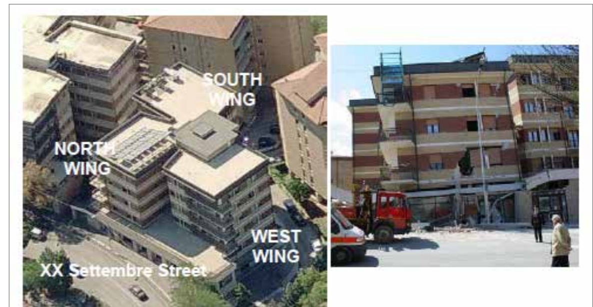
Figure 1. Casa dello Studente. Left: aerial view of the building before collapse. Right: the soft-story of North wing, view from XX September Street.
