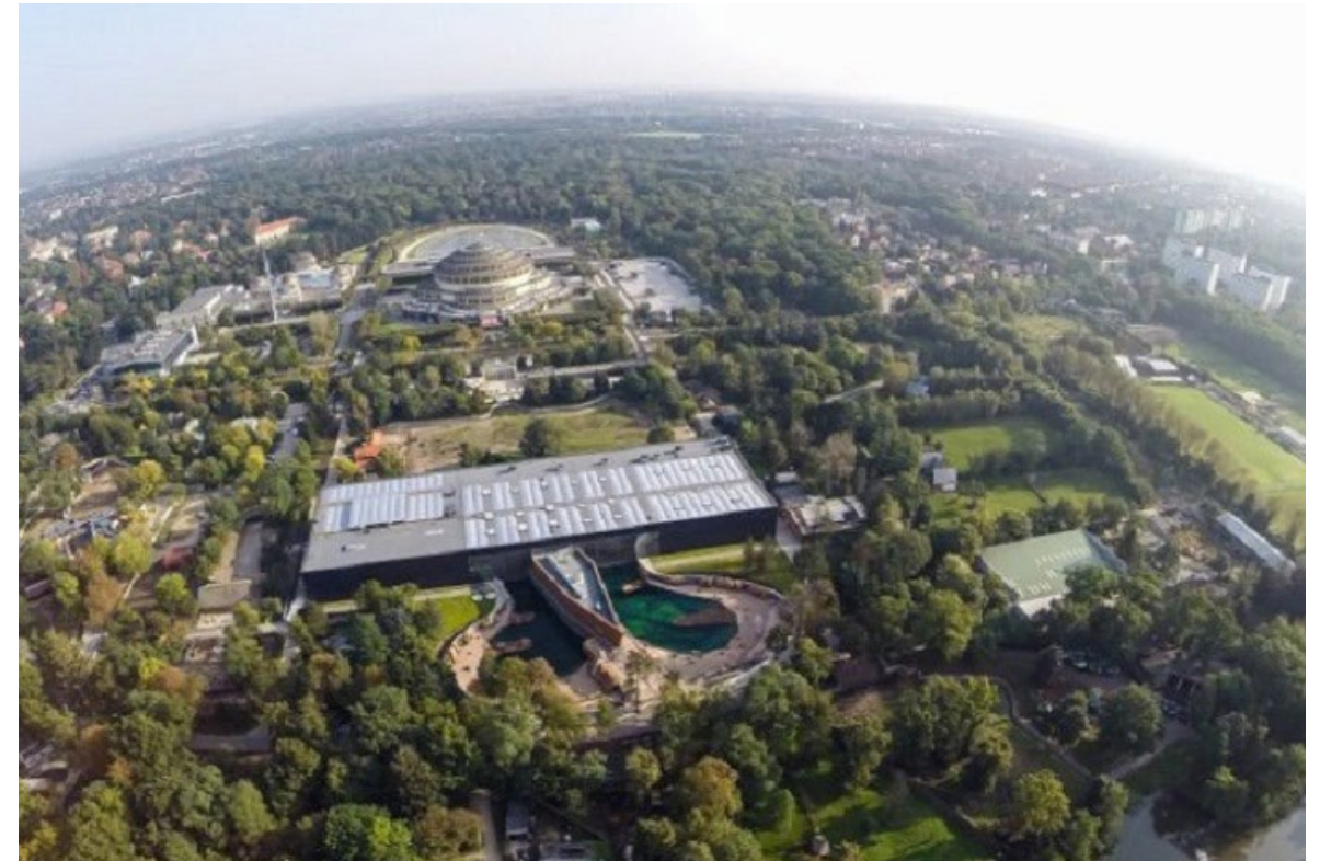
Vista aerea del complesso_Photo on o bryla.pl by ArC2
